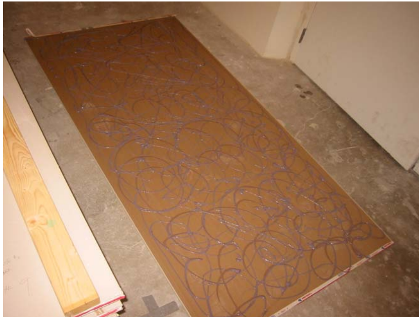
Figure 1: Random application of 56 oz. of QuietGlue Pro to a gypsum panel.
