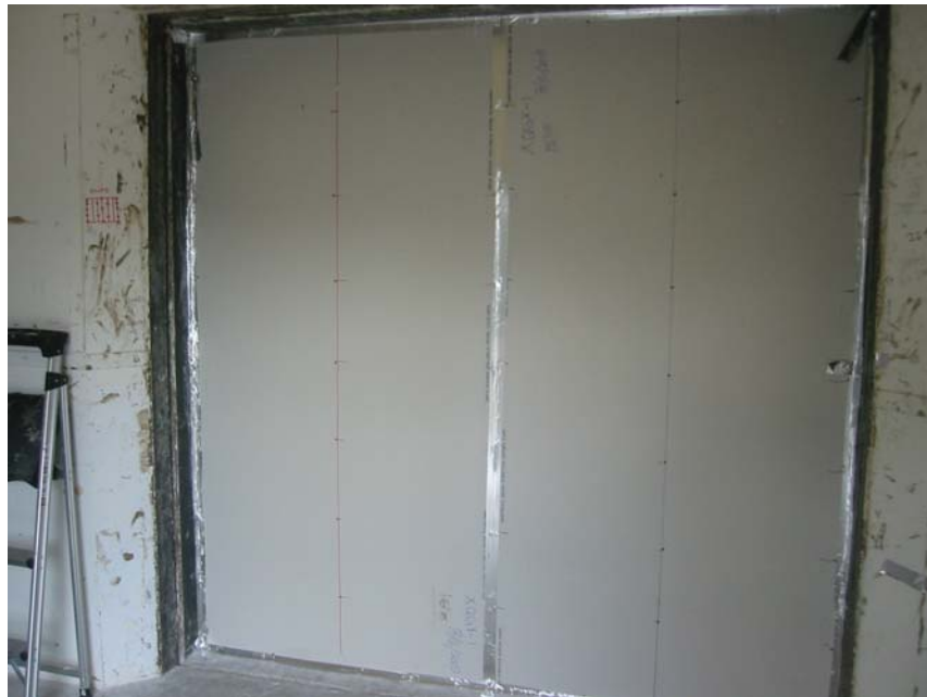
Figure 3: Representative installation viewed from source room side.
