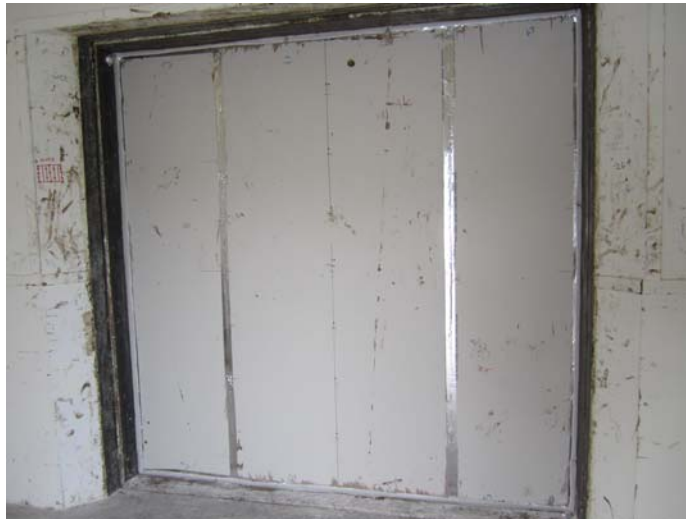
Figure 3: Source room side sheeting installed and sealed
