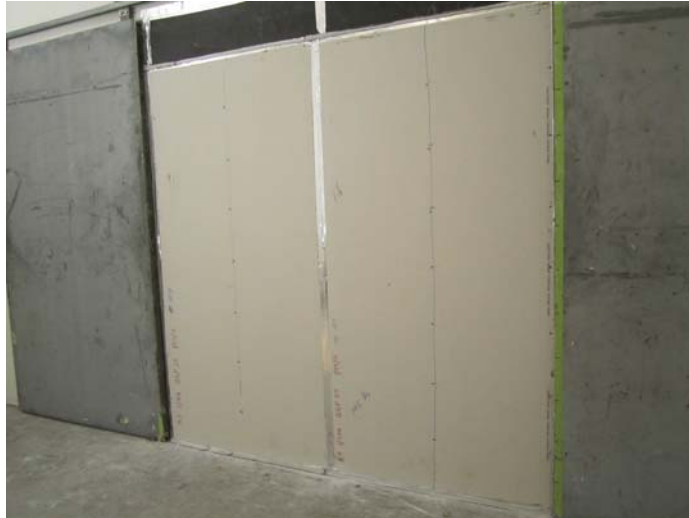
Figure 4: Receiving room side sheeting installed and sealed
